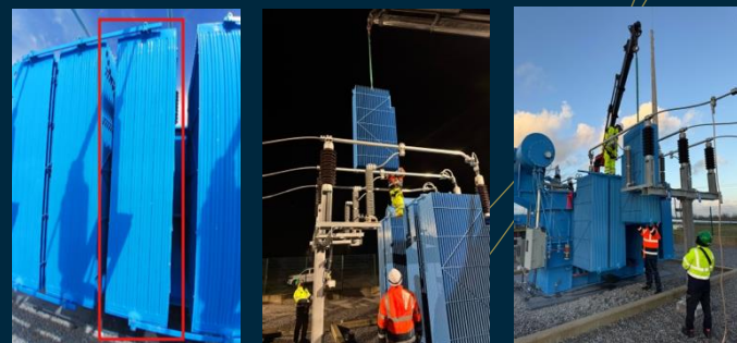
Mina-Tó – Transformer Leakages repair
