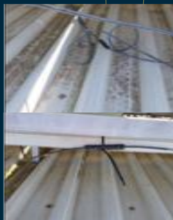
Sol de Tilla – MC4 connector Replacement and cable tie
